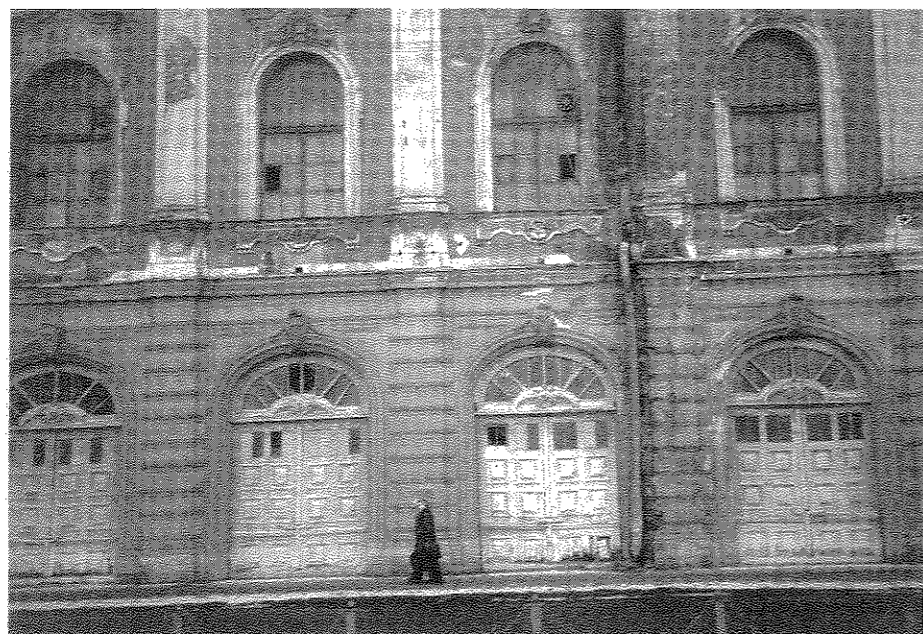
These former imperial stables are now dilapidated and occupied by auto repair workshops.
